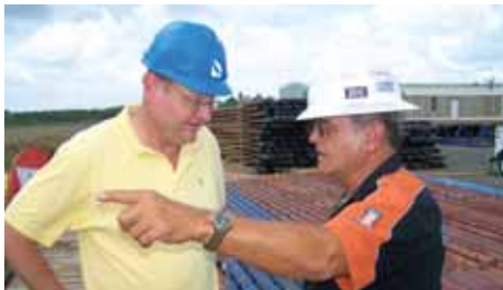
Jim Pitts (left), AGL Resources vice president of midstream operations, and Chief Inspector Wayne Marceaux inspect progress at the Golden Triangle Storage plant site.
