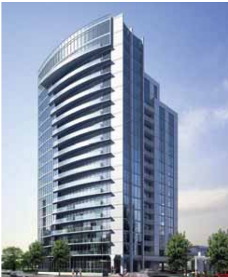
Atlanta Gas Light's partnership with Tivoli Properties, Inc. at its "Mezzo" project allows customers to use natural gas in high-rise buildings.
