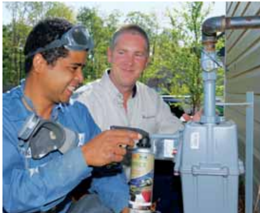
Ken Born, Operations Foreman of Atlanta Gas Light (AGL), observes Robert Williams of Integrated Construction Management (ICM) inspect a gas meter. Through the Supplier Diversity Business Development Program, AGL worked with ICM to help them grow their business and provided field training on identifying whether a meter needs painting and properly painting a meter.
